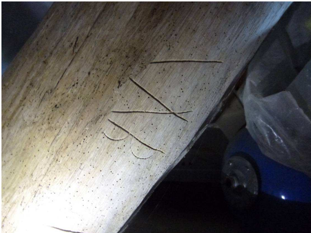
Unusual lumber mark on the west principal rafter of truss T2
