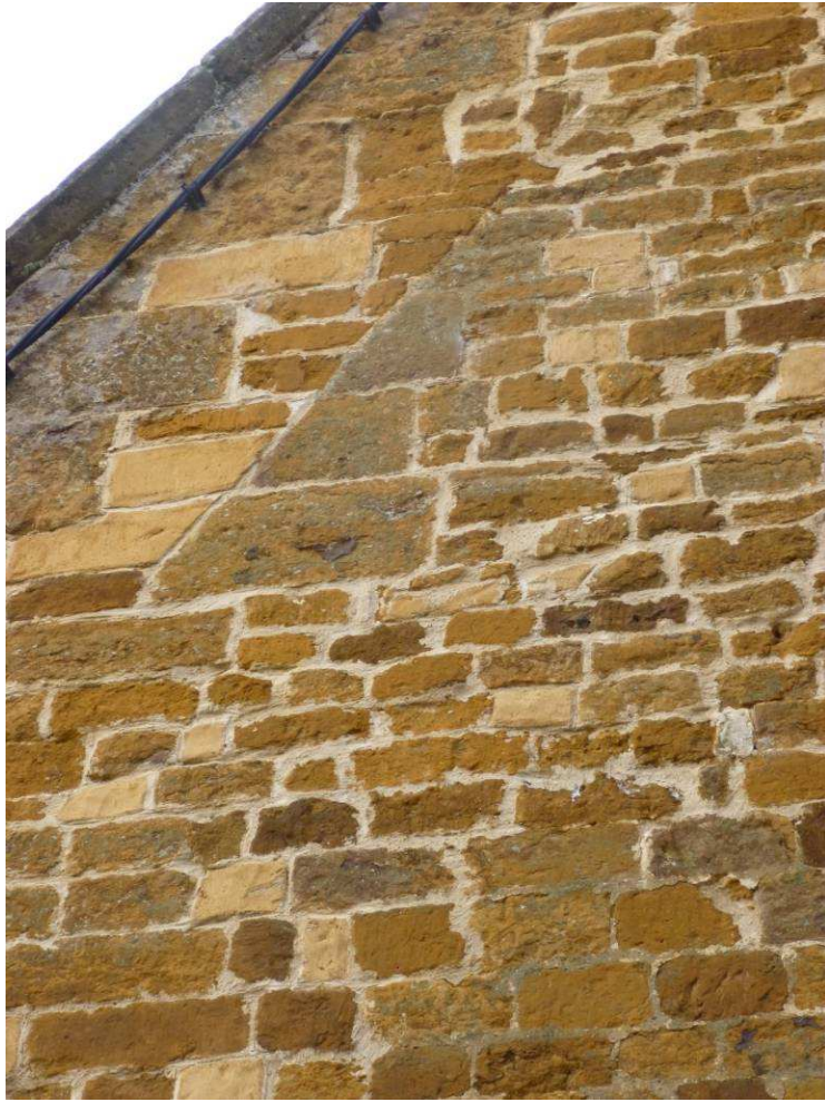
Line of previous gable visible to east end
