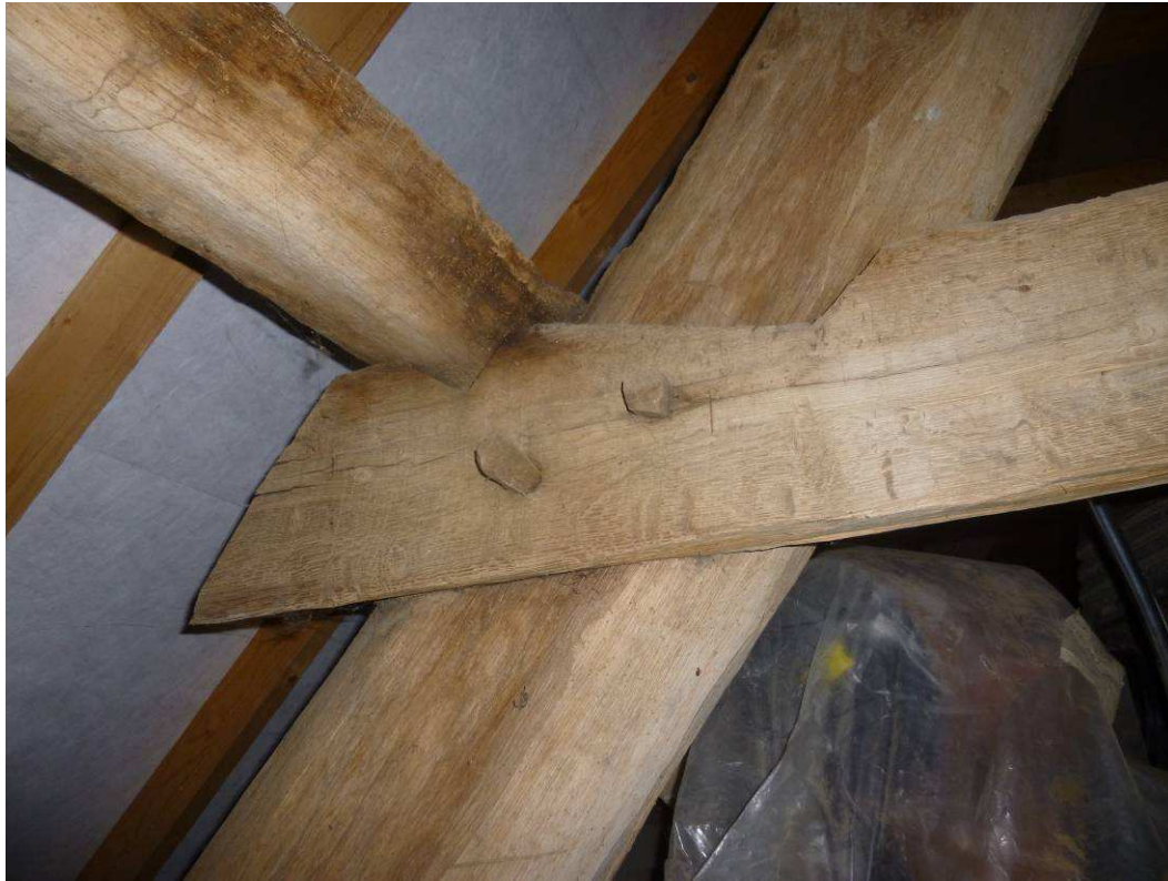
Lower collar joint to truss T2, south side
